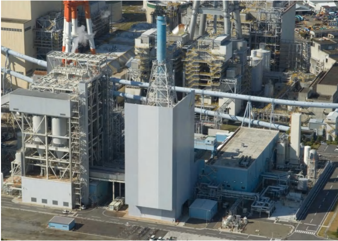
250MW CGCC(Coal Gasification Combined Cycle) Thermal Generation Plant
