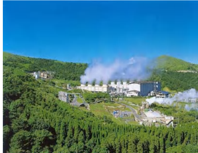
Geothermal Power Plant
